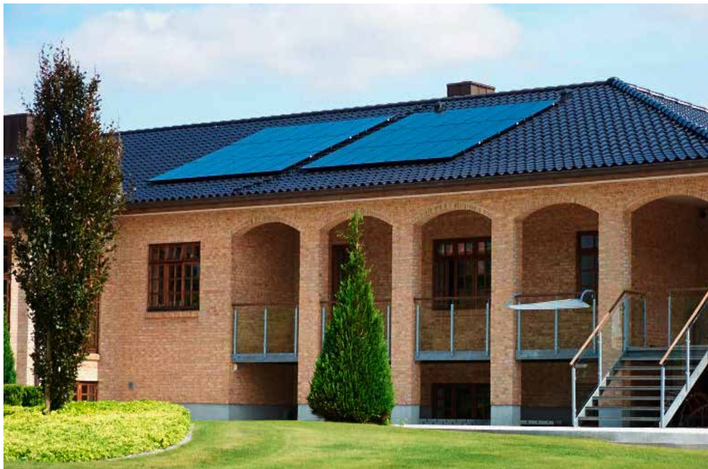
Fig. 1 – Thin-film modules with 6 kWp on a private home (Photo: KlimEnergi A/S).
