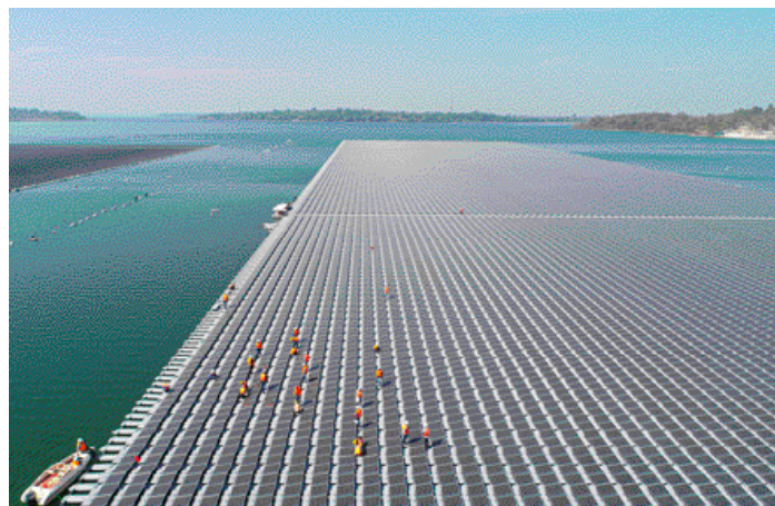
Fig. 1 - The 45 MW world's largest floating PV system, as part of the Hydro-Floating Solar Hybrid Project at Sirindhorn Dam, operated by the Electricity Generating Authority of Thailand (EGAT). This project will hybridize the FPVs with the hydropower dam to increase efficiency of the system (Photo: EGAT).
