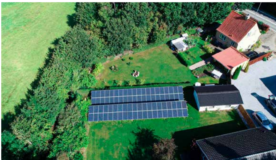
Fig. 2 - Vester Skerninge, Fyn. Privately owned with 20 kWp PV plant with a 16 kWh lithium battery (Photo: KlimaEnergi A/S).
