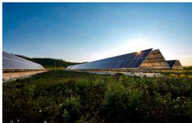
Fig. 1 - The Old Crow Solar Project, a 940 kW system installed by the Vuntut Gwitchin Government in Old Crow, Yukon, 128 km north of the Arctic Circle (Photo: Solvest Inc.). 3
