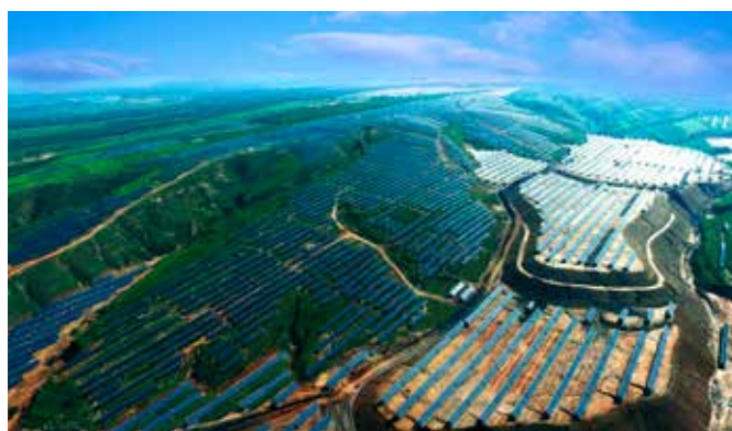
Fig. 3 - Baicheng PV Project (Photo: SUNGROW).
