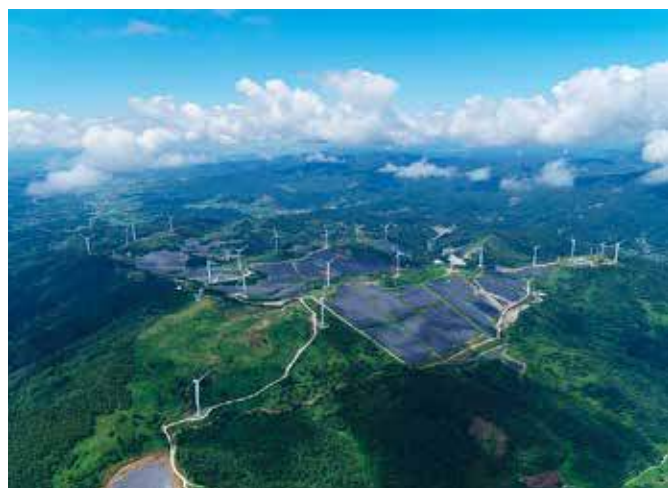
Fig. 2 - 94 MW PV system at Yeongam-gun, Jeollanam-do, Korea.
