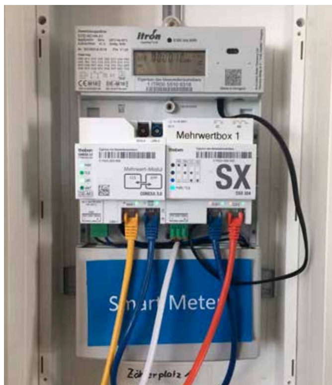
Fig. 2 - Smart Meter Infrastructure providing secure bidirectional communication with decentralized energy systems. The Smart Meter is shown in the background. The Smart Meter Gateway (secure router) is the Connexa 3.0 CX component on the left side. The SX-module on the right side hosts the secure communication with the solar inverter, storage or e-charging wallbox (Photo: © THU, Theben AG).
