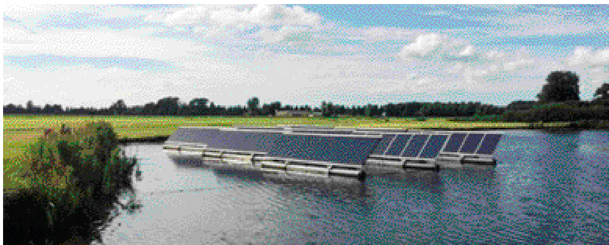
Fig 2 - Floating Solar, ZOGRUNN project (Photo: RVO).
