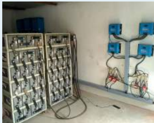
Figure 30 Battery bank and maximum power point tracker (MPPT) in Phori village
