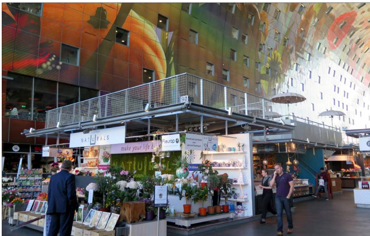
Photo 6.1 Densification: housing on top of a market square: Market Hall, Rotterdam, designed by MVRDV; artwork by Arno Coenen
